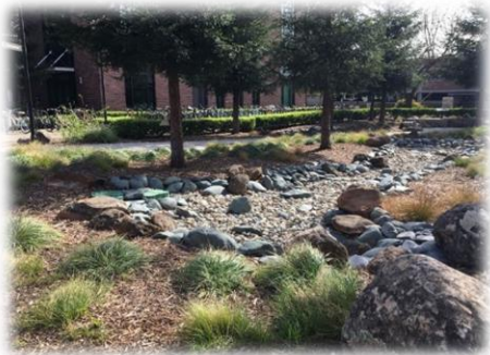
A campus bioswale, a biological, storm-water contaminant filter
